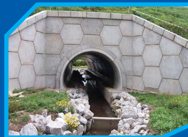
An example of mammal ledges on a culverted stream under a road (Source: NRA)
